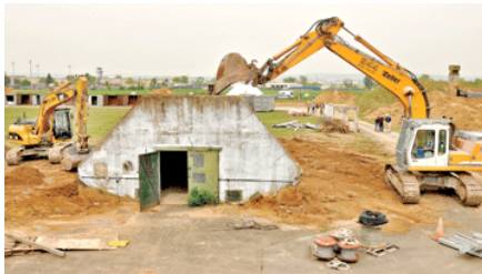
Demolition of old WAA storage bunkers
